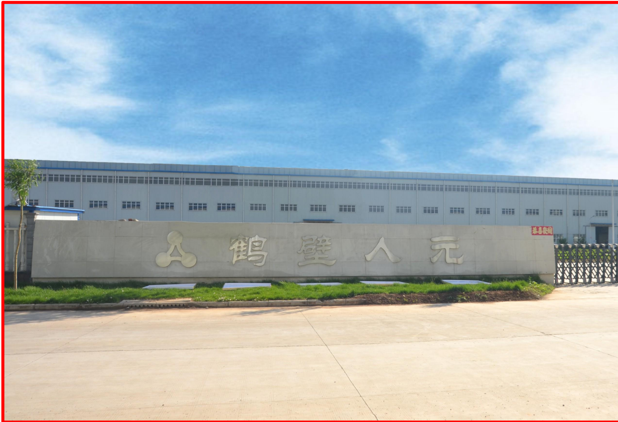
Main gate of equipment plant
